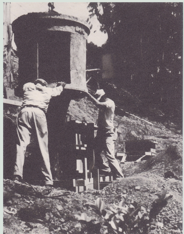
Construction at 6624 Saroni Dr
